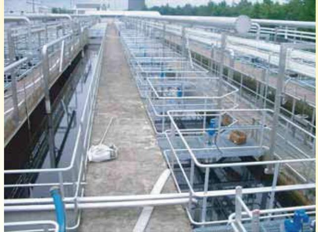
Anaerobic/aerobic reactor tanks, 93 units, 55 m<sup>3</sup>, 0,55 kW. Sweden
